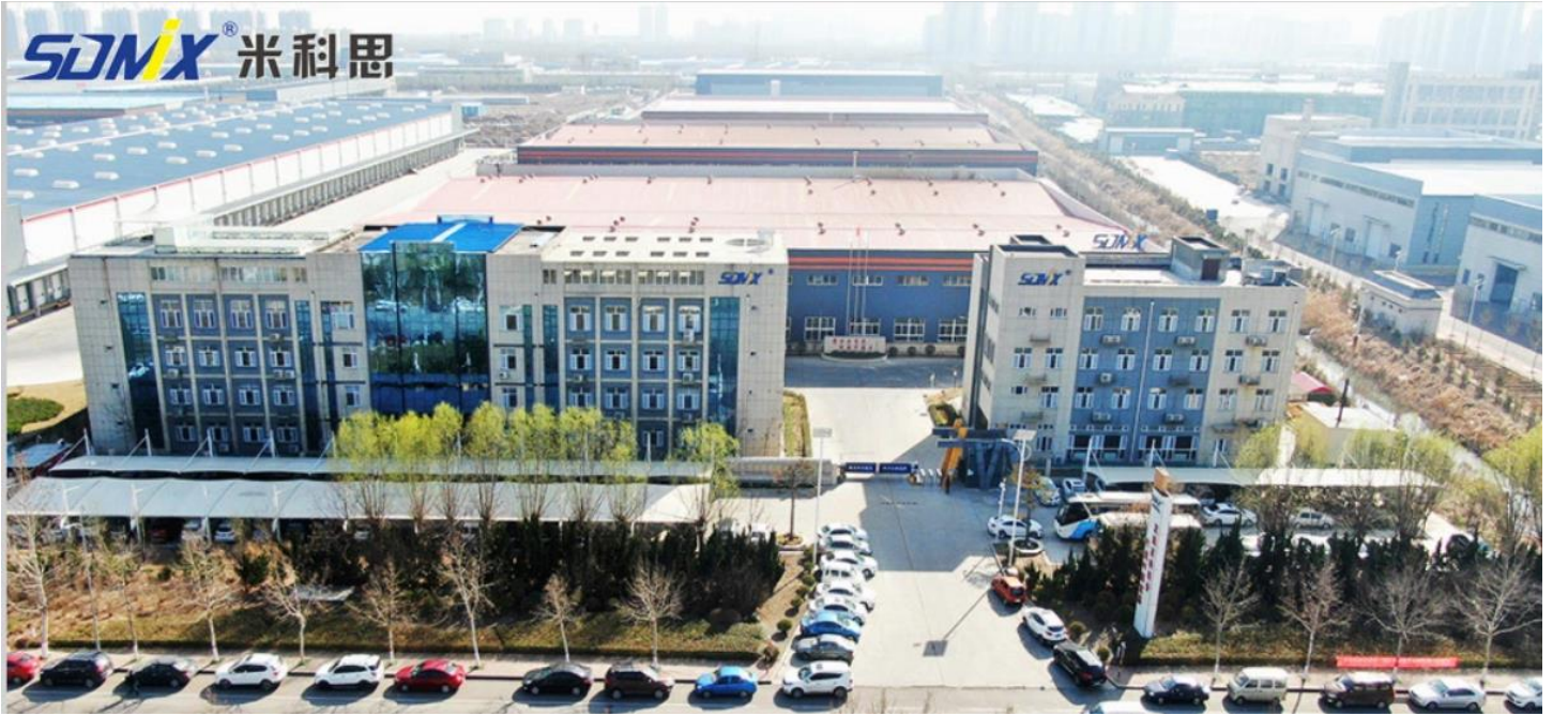
SDMİX MERKEZ FABRİKA, Şantung Eyaleti-ÇİN / SDMİX CENTRAL FACTORY, Shandong Province-CHINA
